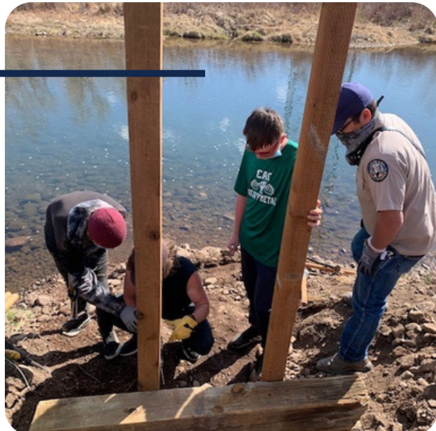
Creating Stabilizer for Eroded Area
